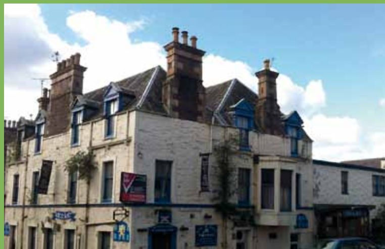
The Strathearn Hotel, one of Crieff's many derelict and vacant buildings
