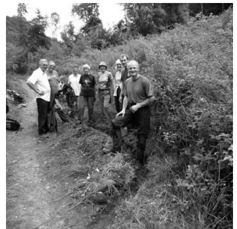
Volunteers working on the path at Trowan
